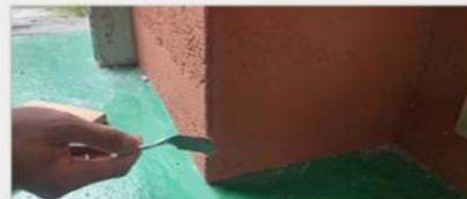
Flatten with a scraper
