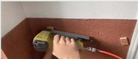
Fixing with pneumatic nails
