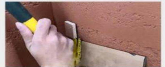
Pull out the air nail
