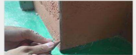
Caulking of Begonia Corner
